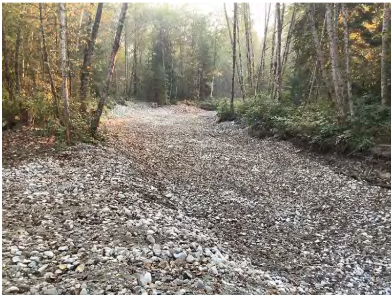
Downstream channel work
