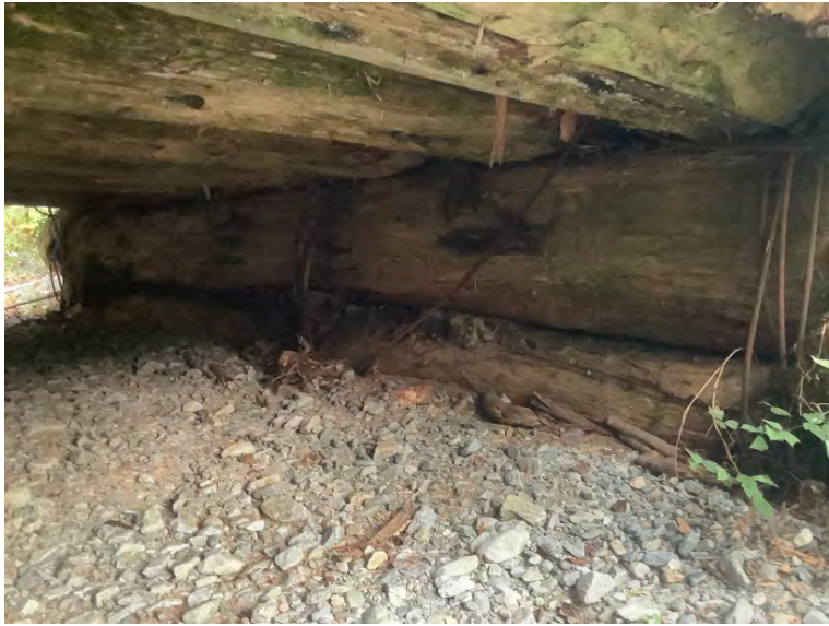
Left Bank Abutment when facing downstream
