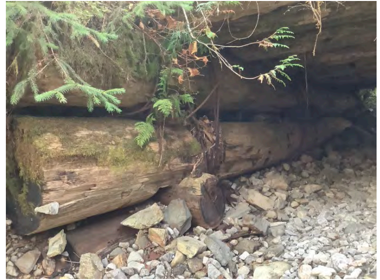
Right Bank Abutment when facing downstream
